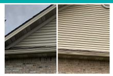
7. Gutters: Aluminum - Gutter not properly sealed in front, Recommend repair
