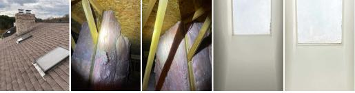
7. Marginal Flashing: Metal - Flashing not sealing properly on side of home, recommend repair
